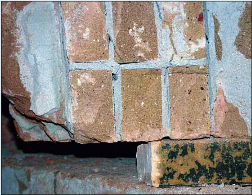
The cracks at the brick/mortar interface are the result of the difference in linear expansion coefficient.
